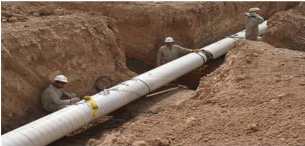
Construction of Fire Fighting system in Al Haritha Power Station
