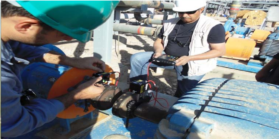
Pump Alignment By Using Laser Method
