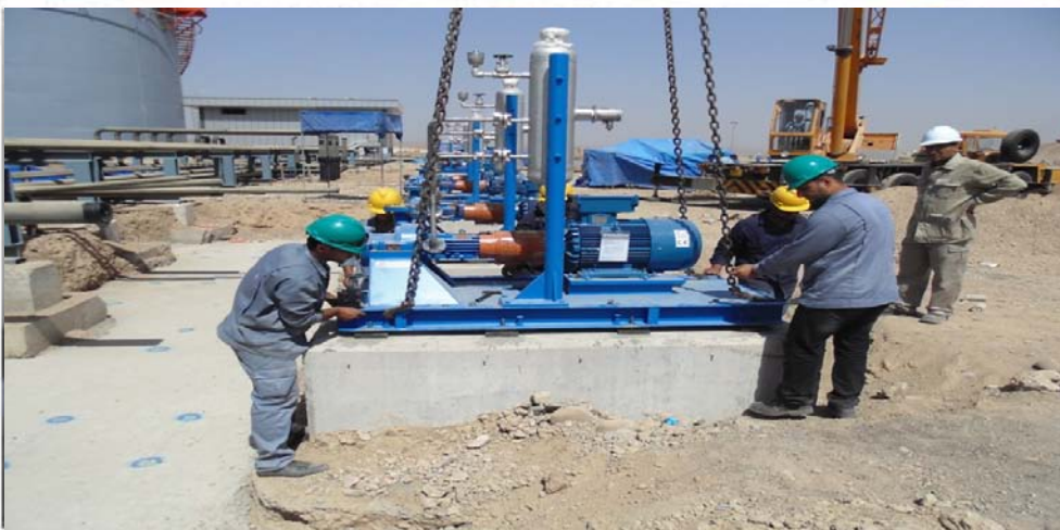
Pump Installation Completion
