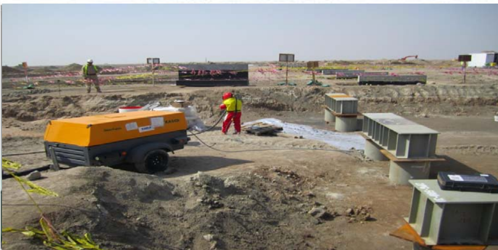
Sandblast Equipments With Protection Safety Mask For Sandblast Activities
